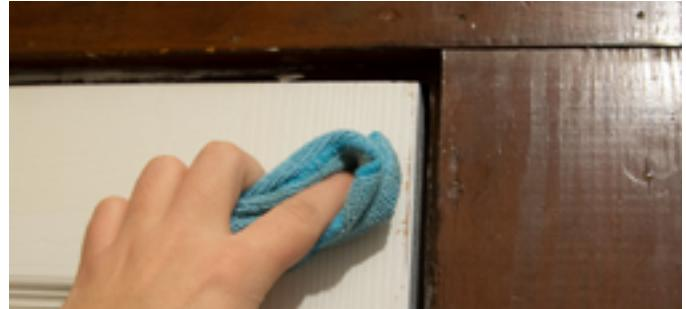
**Step 4:** Place one sensor on the door well. Ideally the larger sensor should be in the door well. In some situations you may have to place the smaller sensor in the door well. Press and hold the sensor on the door well for 10 seconds to ensure a strong connection.
